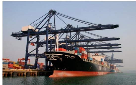
STS container crane
