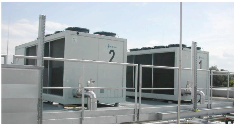
Rhoss, Italy. New motor starting solution from ABB reduced inrush currents of scroll compressors by 60 percent.
