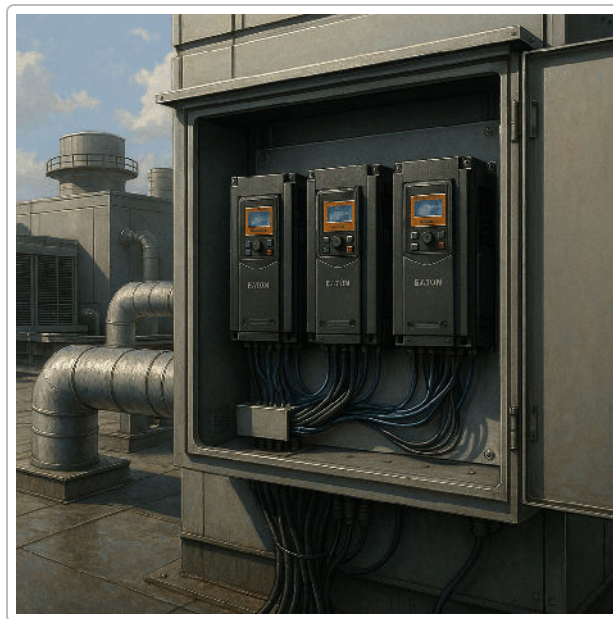
Figure 2: Three Eaton PowerXL VFD units installed on rooftop HVAC fans. By modulating fan speed to maintain target building pressure and airflow, such VFD retrofits can eliminate inefficient throttling methods. In one documented retrofit, a 40 HP fan VFD saved ~35,000 kWh per year (≈$4,100) and improved system stability, paying back the investment in ~1.5 years. (Image: Precision Electric, Eaton HVAC case)
